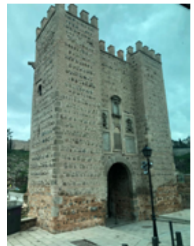
Figure 3: Entrance Gate to the city of Toledo.
